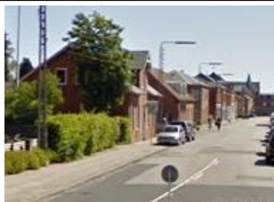
Red brick buildings along Vestergad Street, Haslev, date from the 19 th century and currently are used for shops and residences. Neither structural nor cosmetic damage were allowed.
